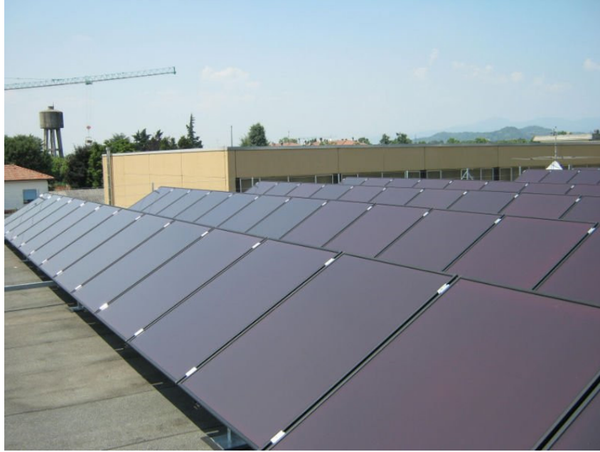
Figure 4 - Thin-Film Amorphous Silicon (Haven Hill, 2018).
